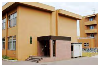
明誠寮(男子寮) Meisei Dormitory (male dormitory)
