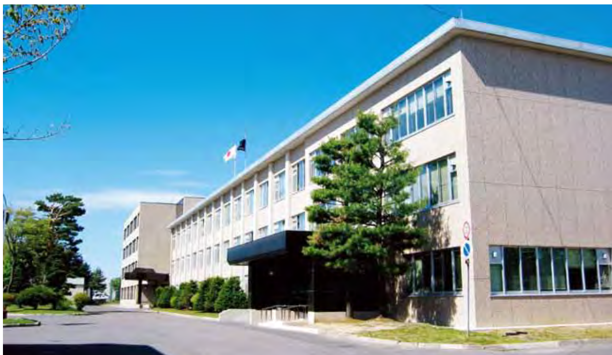
校舎 School Building
