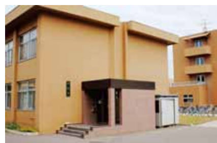
明誠寮(男子寮) Meisei Dormitory (male dormitory)
