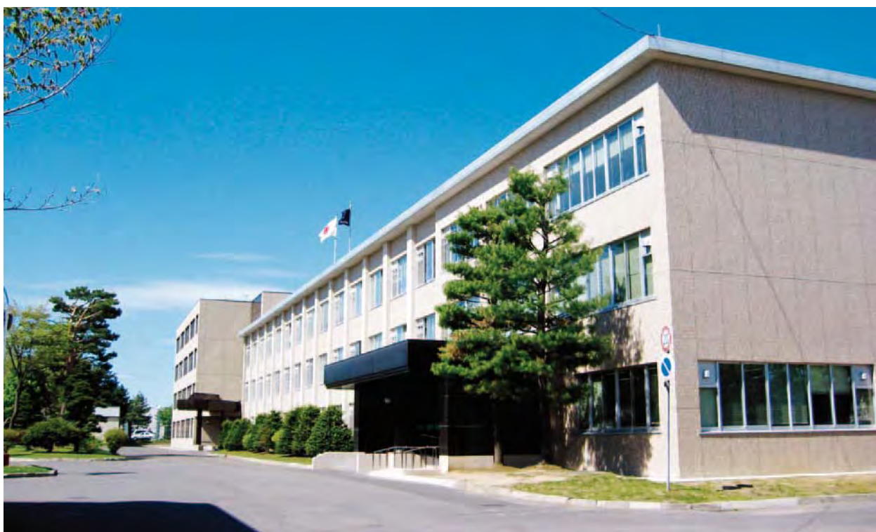
校舎 School building
